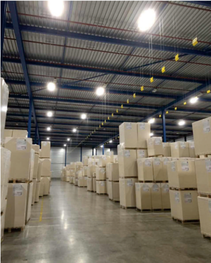
Date: June 18th, 2016 Product: MagicSquare high bay 150W (30*70 degree) Application: Warehouse Country: Netherlands
